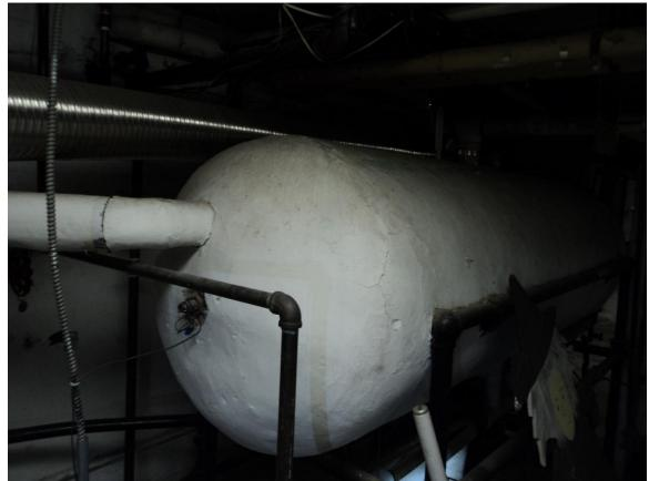
Asbestos was also noted around the hot water tank in the basement of the house.
