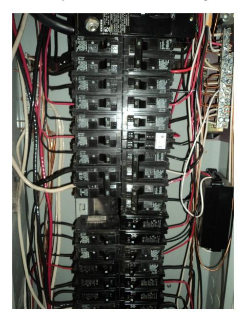
There was a Leviton electric box located in this panel that should be moved outside the main electric panel box at this time.
