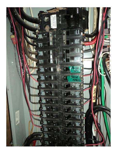
The 2<sup>nd</sup> main electric panel was also located in the basement on the rear wall on the right. This panel was a 200 amp panel with 31 breakers. At the time of the inspection
