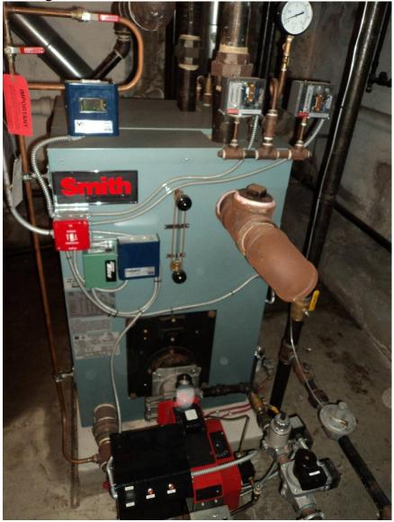
GENERAL VISUAL CONDITON: Good RECOMMENDATIONS: Recommend having the unit serviced and maintaining a service contract. The heating system was **not** working at the time of the inspection. This system needs to be up and running and properly checked. All radiators in the house need to be tested.
