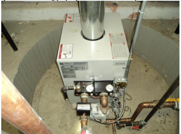
Recommend having the over pressure relief valve on the hot water boiler properly piped at this time as the pipe should have no threads at the discharge.
