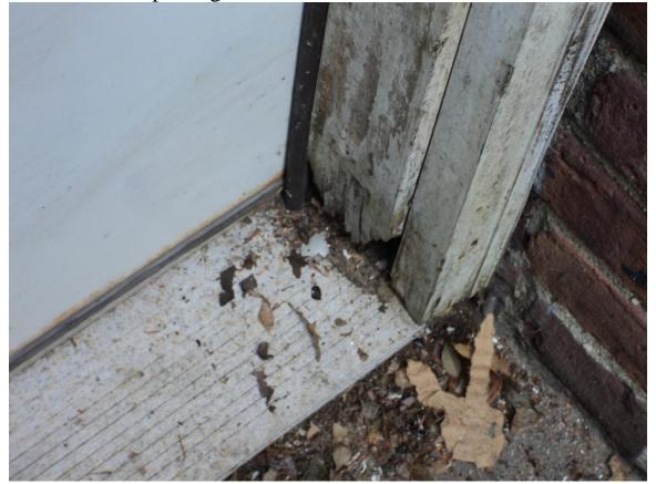
Recommend replacing the rotted wood at the base of the basement entrance door.
