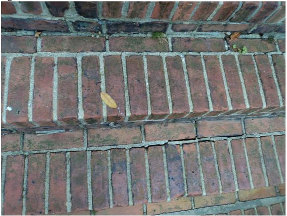
Recommend re-pointing the brick work around the patio on the far left side. There was also water seepage into the basement in this location and the ceiling needs to be opened for a further investigation in this area due to water damage to the main header in this location of the laundry room below.
