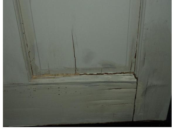
Recommend replacing the rotted door leading to the 2<sup>nd</sup> floor of the garage.
