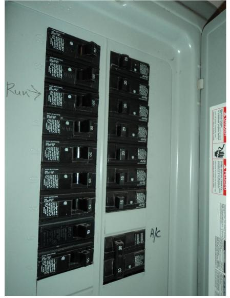
The electric in the pool house was fed from the main house. This panel is a 125 amp panel located in the rear of the pool house with 17 breakers.
