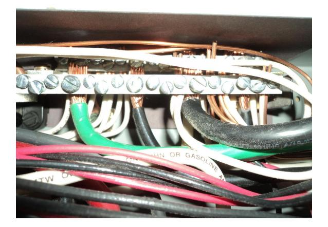
Install knockout covers where missing in this electric service panel.
